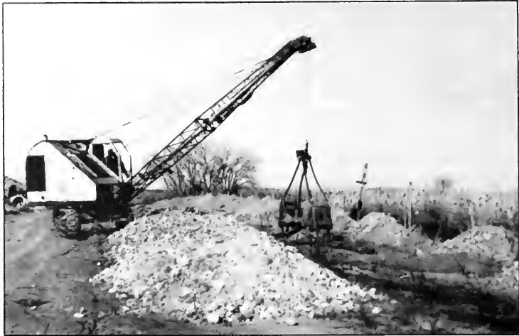
Figure 12.5. Dragline digging deep north drainage trench, 1946.
